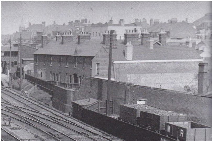
Sundown Place to the right of the railway line. Ilford To Shenfield David Brennand, Middleton Press 2002
