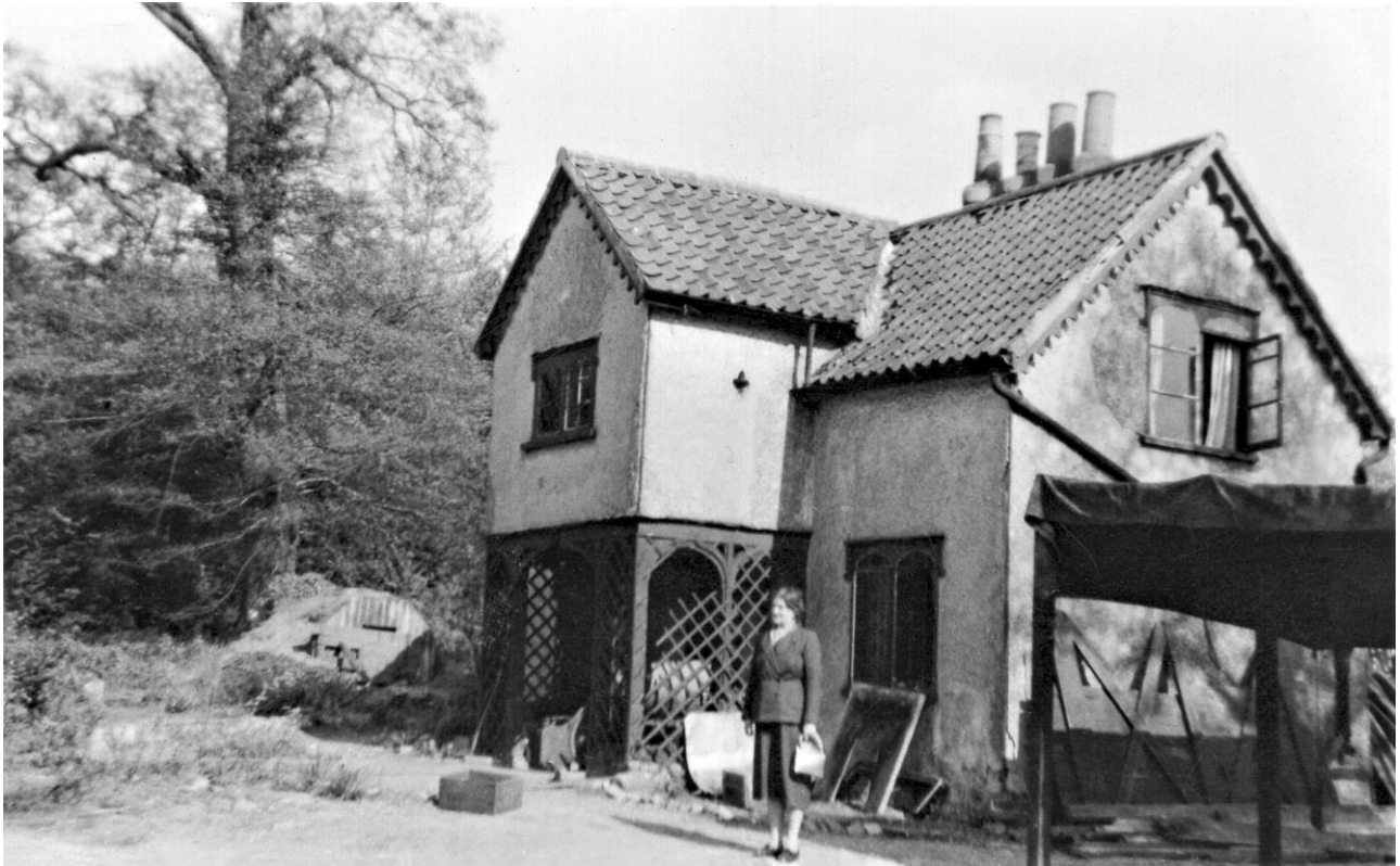
Image 13. Claybury Lodge in the 1950s. By this time, the thatched roof had been replaced with tiles and the first-floor balcony filled in. Just beyond the building can be seen a wartime Anderson air-raid shelter.
