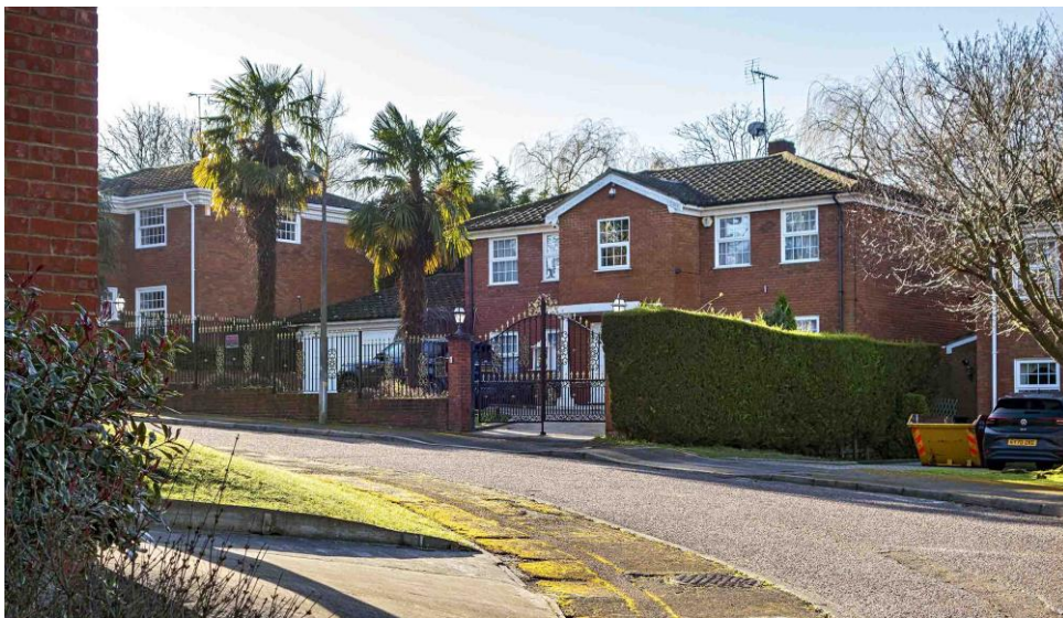
Image 17. Here stood Claybury Lodge from 1800/1801 until 1973 when it was demolished and replaced by these houses in Audleigh Place, as seen in 2022.
